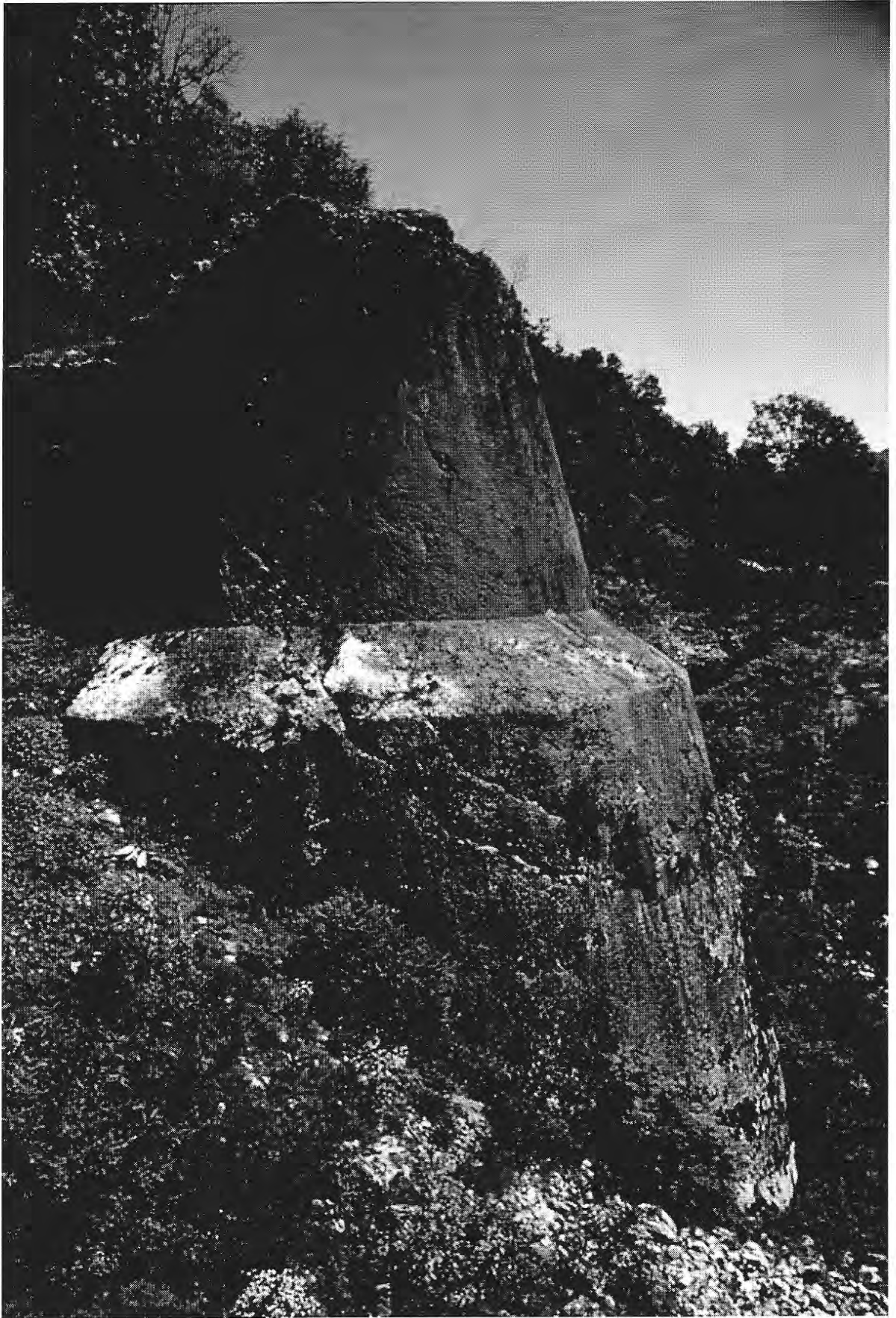
Fig. III.18.a. "Tenaglione verso Stura" cut into the limestone, situated east of the Bastion of Saint Ignatius (photo G. Padovan).
